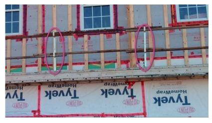
The Featherlite Stanchion post allows the installtion of the Featherlite Platform across a significantly long span. Use of these posts is shown in the above photo. The posts are highlighted by magenta markings.
