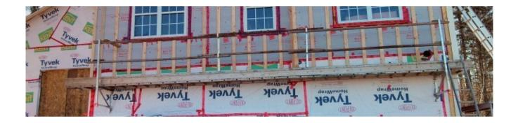
Using the certified Featherlite Platform allows a maximum span of tweenty eight feet or 8.5 metres (pending) between all the platform Brackets.
